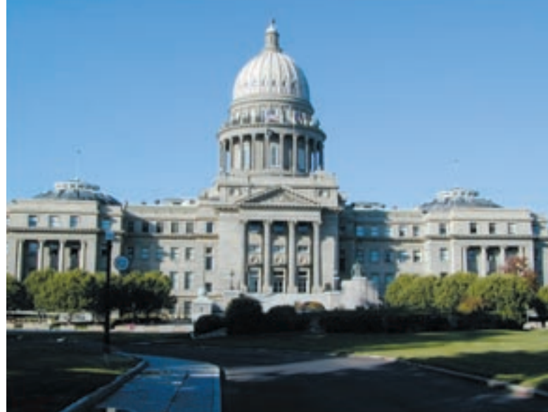
The Idaho State Capitol Building in Boise is heated by the city geothermal district-heating system. PIX13100 NREL
