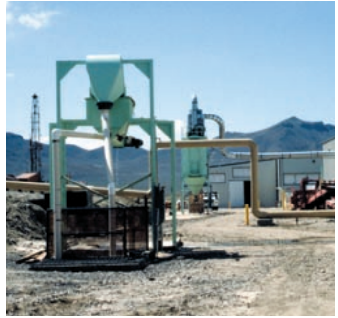
Geothermal energy is ideal for dehydration operations (onions and garlic), as seen in Empire, Nevada.
